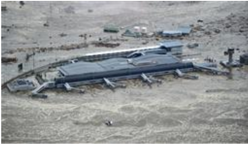
Sendai air port damaged by the tsunami as of March 13th
