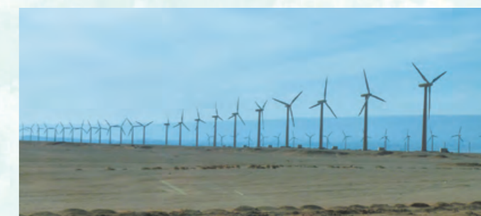
Zafarana Wind Power Plant Project (120 MW) in Egypt supported with Japan's ODA loan (Photo by JICA)
