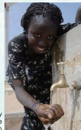
Water tap constructed by Japan's assistance (Photo by JICA/Kenshiro Imamura)
