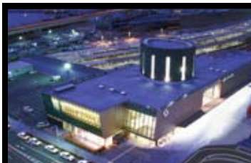
Hakodate Station © Hokkaido Nikken Sekkei Ltd.
